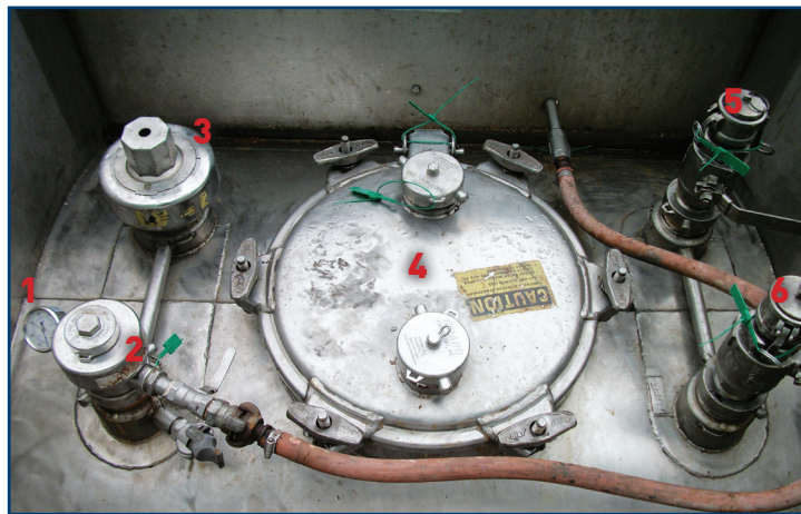
The above photo points out the top fittings of a Cargo Tank Trailer: 1) Pressure Gauge; 2) Vacuum Relief Device; 3) Pressure Relief Device; 4) Manway; 5) Vapor Exchange Valves/ Fittings; 6) Airline in from Desiccant Dryer.
