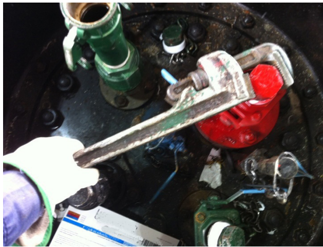
The above photo illustrates proper use of tool to secure the plug.
